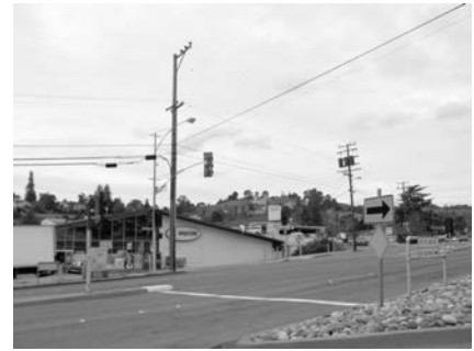
Work with PG&E to underground utilities on major roads in residential neighborhoods, such as here at Lake Chabot Road and Seven Hills.
