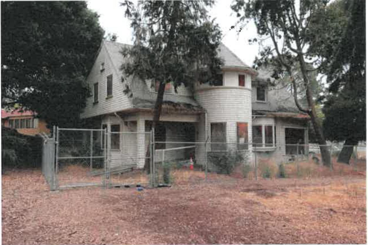
Fig.3 – Superintendent's Residence/Whitecotton Cottage, West side, 2018
