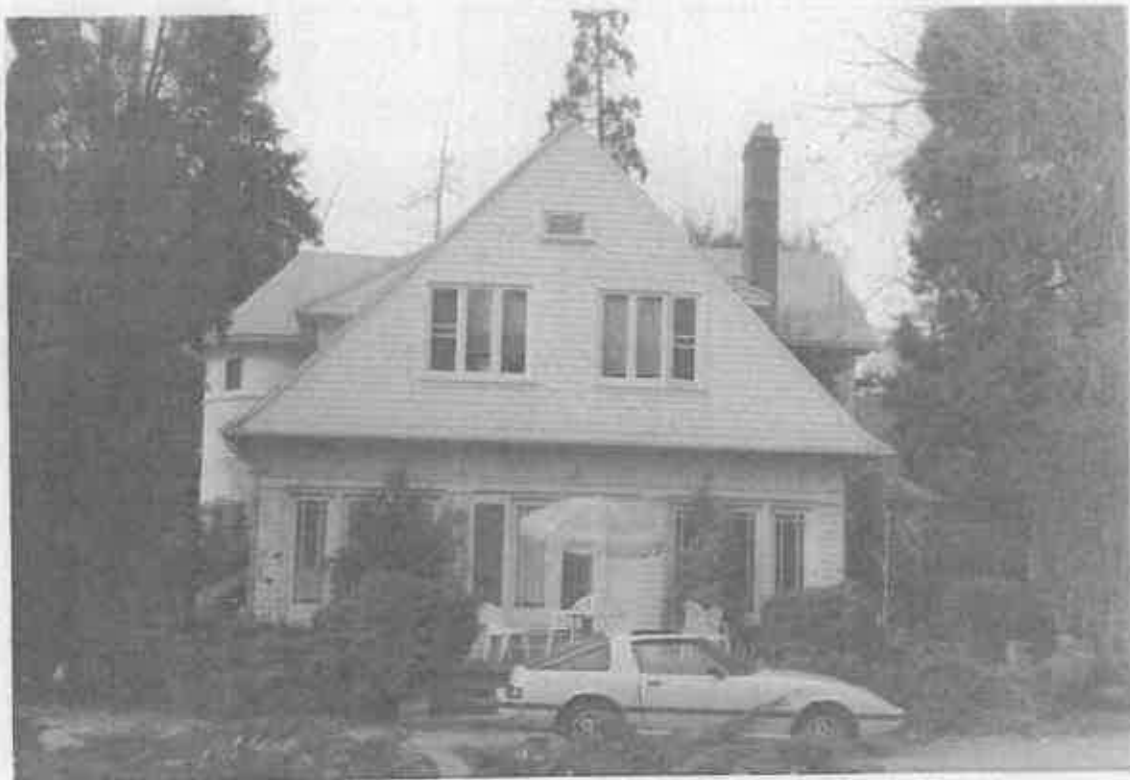
Figure 3. South Elevation, Superintendent's Residence, Fairmont Hospital.
