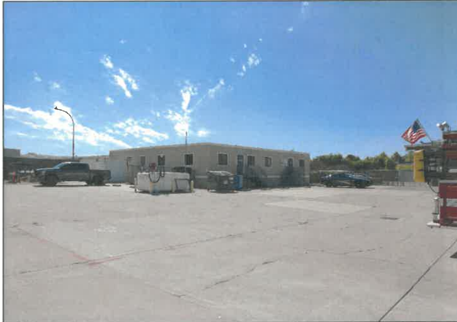
Photograph 10: Contemporary prefabricated building at rear (east) side of property, camera facing southeast, August 15, 2023.
