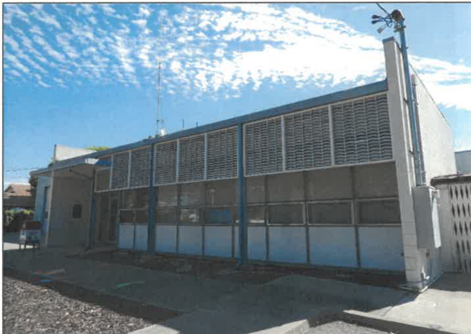
Photograph 5: West façade of office and living section of station, showing curtain wall with sunshades. Camera facing northeast, August 15, 2023.
