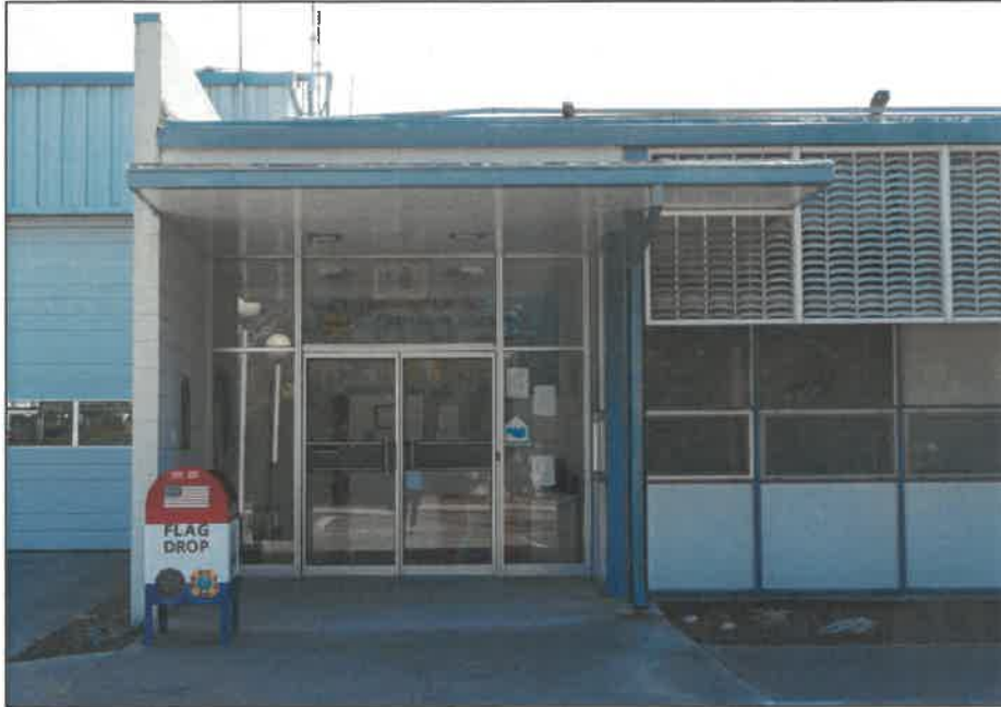
Photograph 4: Main entrance to station on west façade, camera facing east, August 15, 2023.
