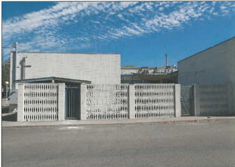
Photograph 7: Concrete-block wall enclosing courtyard and storage area (left), camera facing north, August 15, 2023.
