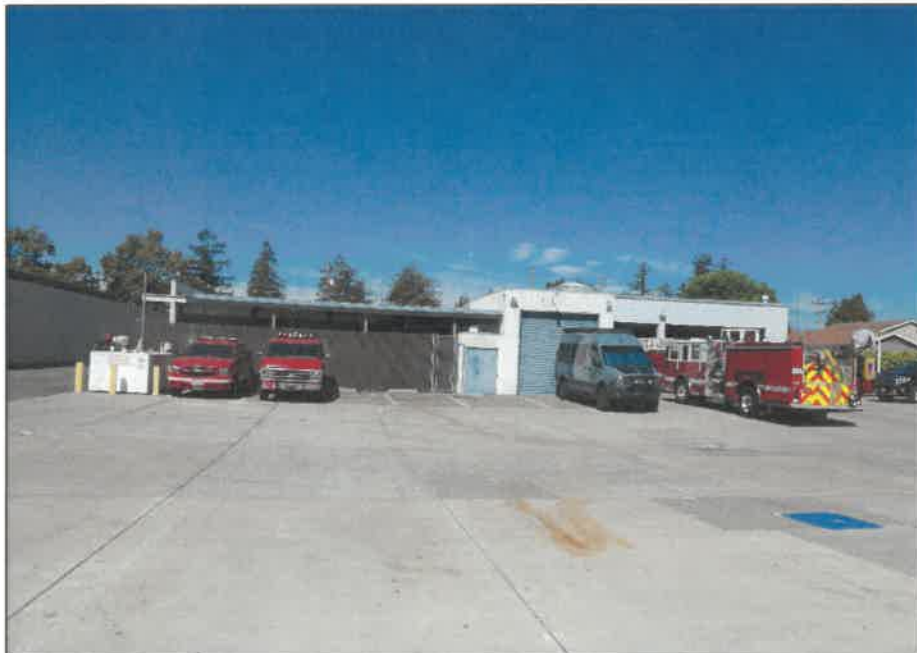
Photograph 9: East side of station showing apparatus section (right), repair shop (center), and enclosed planting area (left), camera facing west, August 15, 2023.
