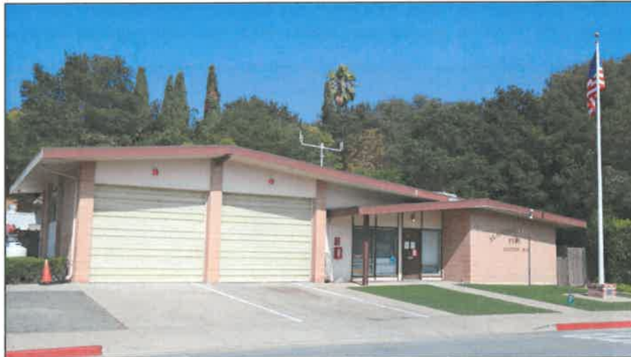
Figure 3: CVFPD Station No. 3 (ACFD Station No. 26), ca. 2020. 16
