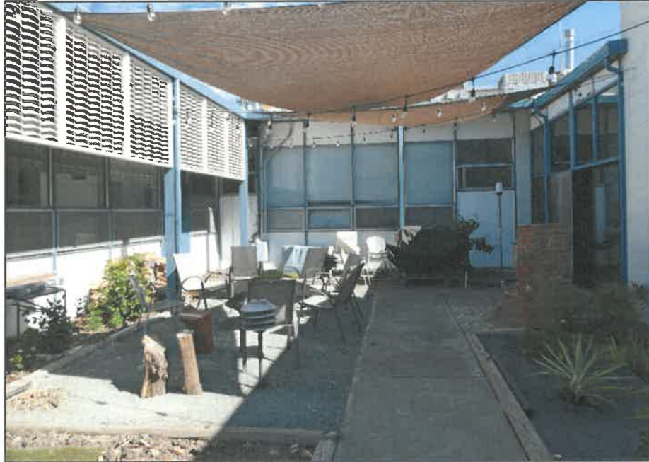
Photograph 6: Concrete-block wall enclosing courtyard and storage area (left), camera facing north, August 15, 2023.
