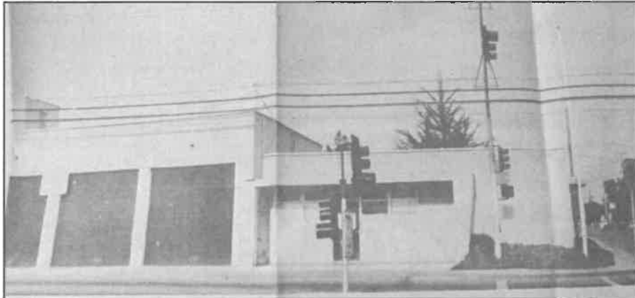
Figure 2: View of the old Station No. 2, constructed in 1953 at intersection of Redwood Road and Heyer Avenue, in 1981. 12
