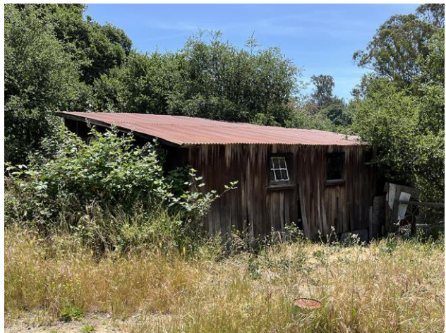
Figure 6. Shed near southeast corner of the property, looking southeast.
