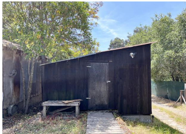
Figure 4. Redwood shed behind house, looking south.
