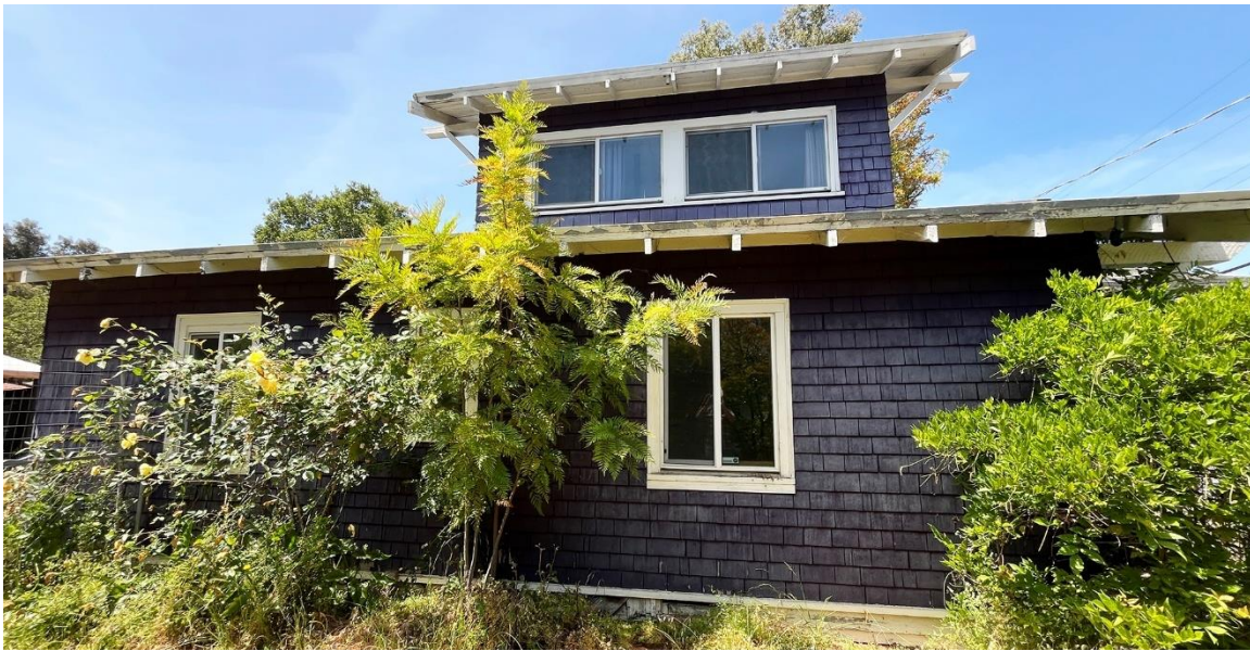
Figure 12. East façade (front portion), looking west.
