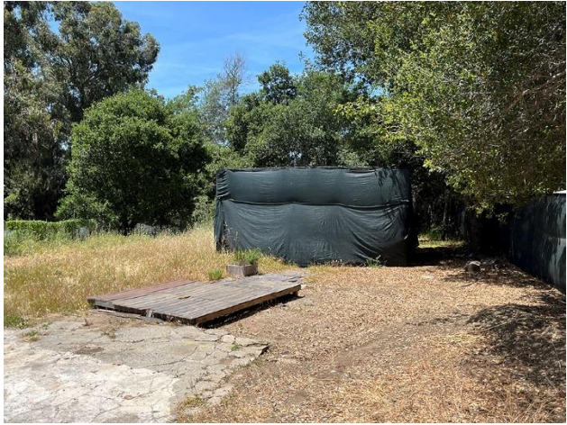
Figure 5. Parking area and garden enclosure, looking west.
