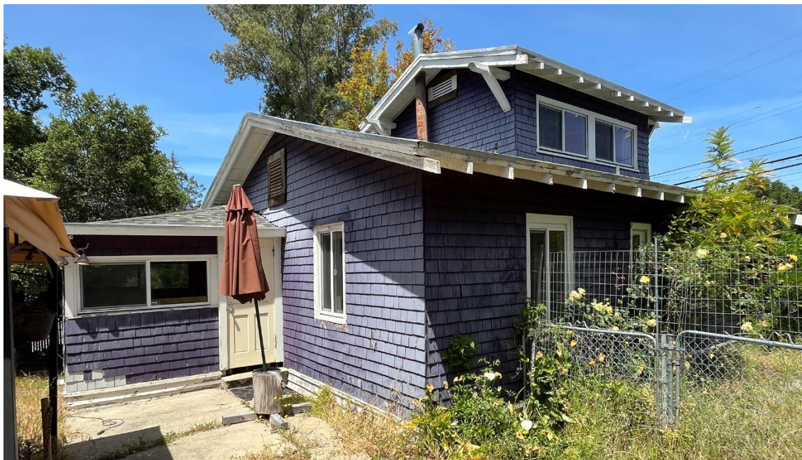
Figure 13. East façade (rear portion), looking northwest.
