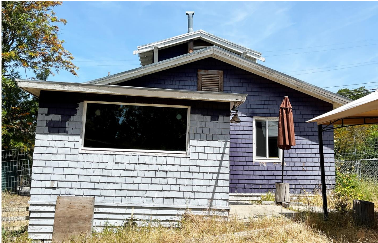
Figure 14. South (rear) façade, looking north.
