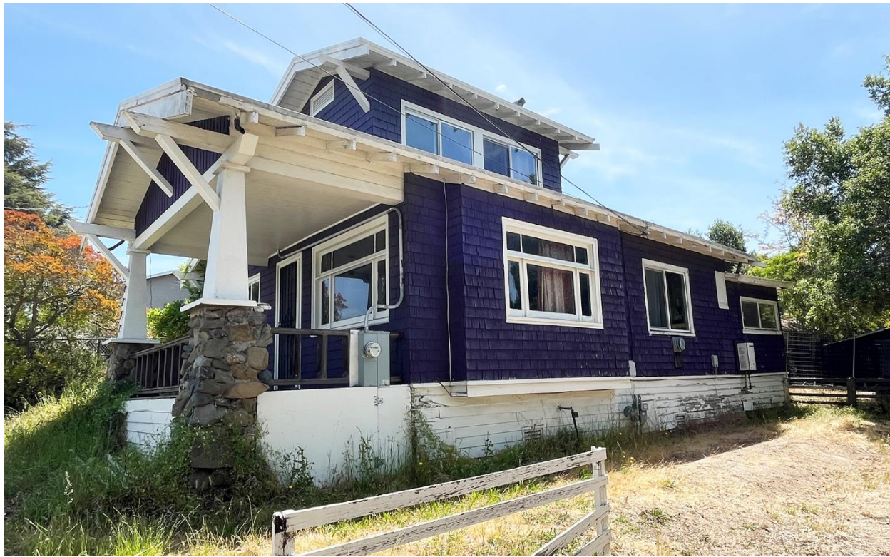
Figure 10. West (secondary) façade, looking southeast.
