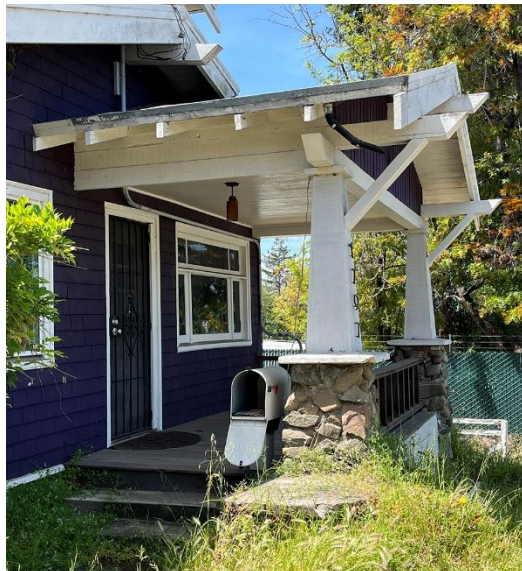
Figure 8. Detail of front porch, looking west.
