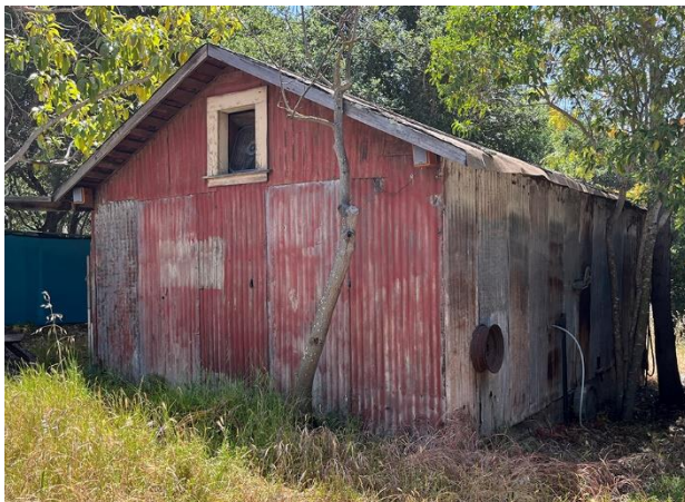
Figure 3. Corrugated metal shed behind house, looking southeast.
