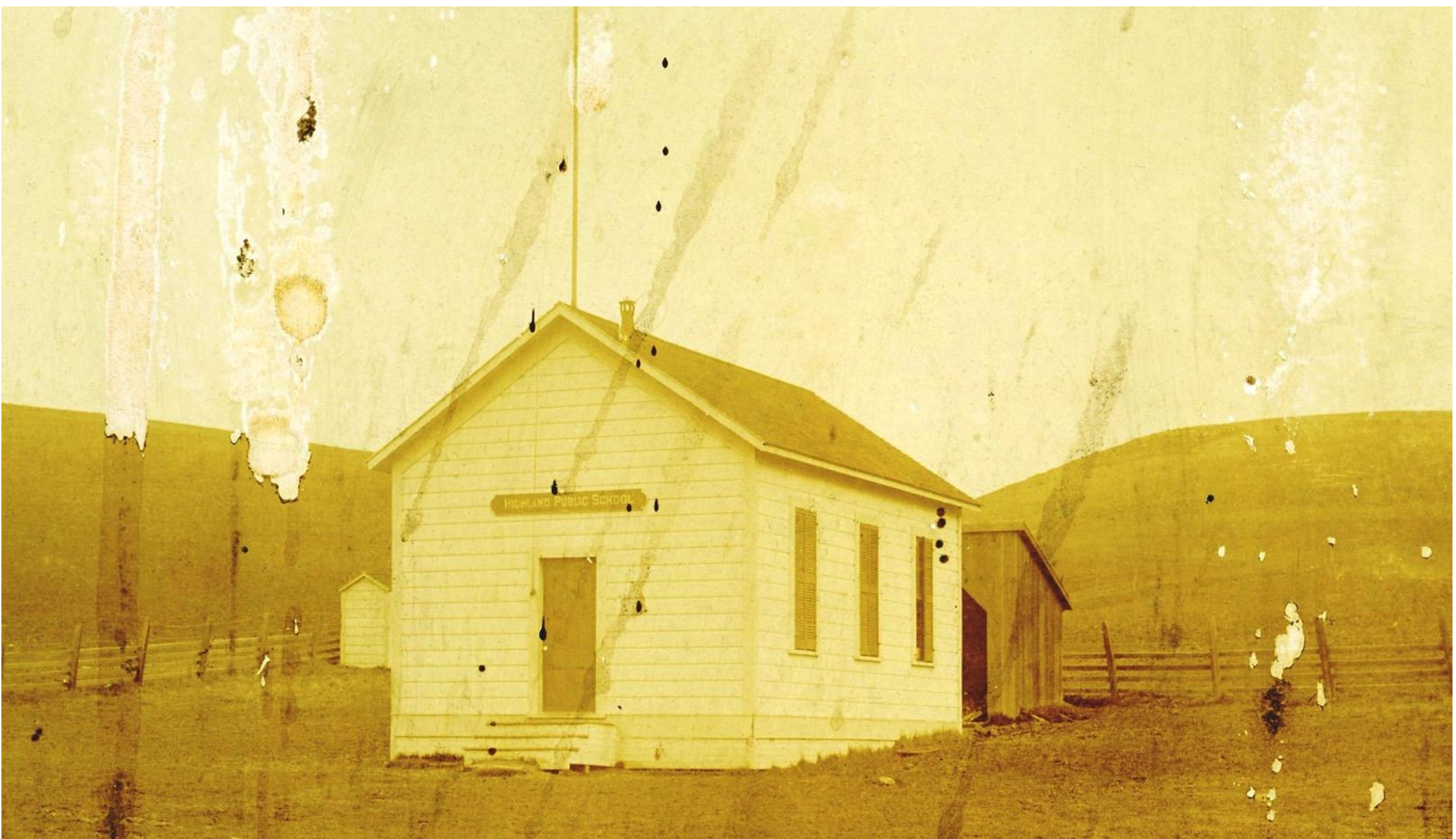
Highland School, Built 1879, N. Flynn Rd, near Sweet Ranch
