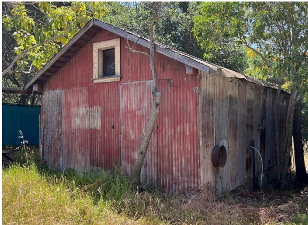
Figure 3. Corrugated metal shed behind house, looking southeast.
