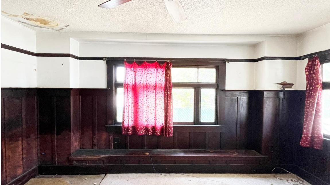
Figure 15. Living room, looking east toward inglenook.
