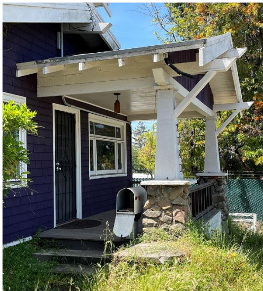
Figure 8. Detail of front porch, looking west.
