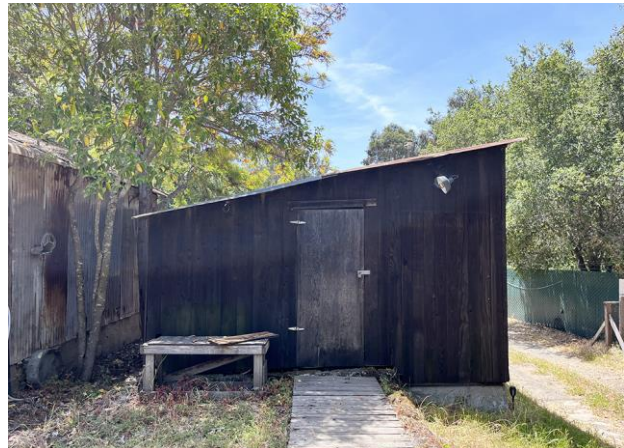
Figure 4. Redwood shed behind house, looking south.
