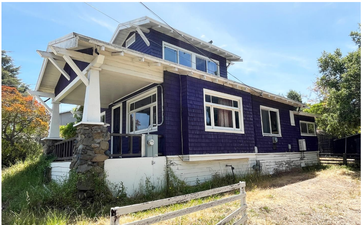
Figure 10. West (secondary) façade, looking southeast.
