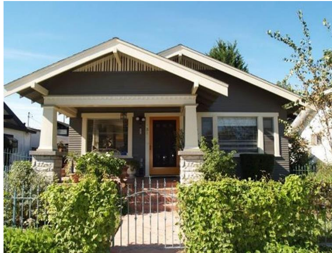
Figure 18. Quintessential California bungalow in Berkeley.
