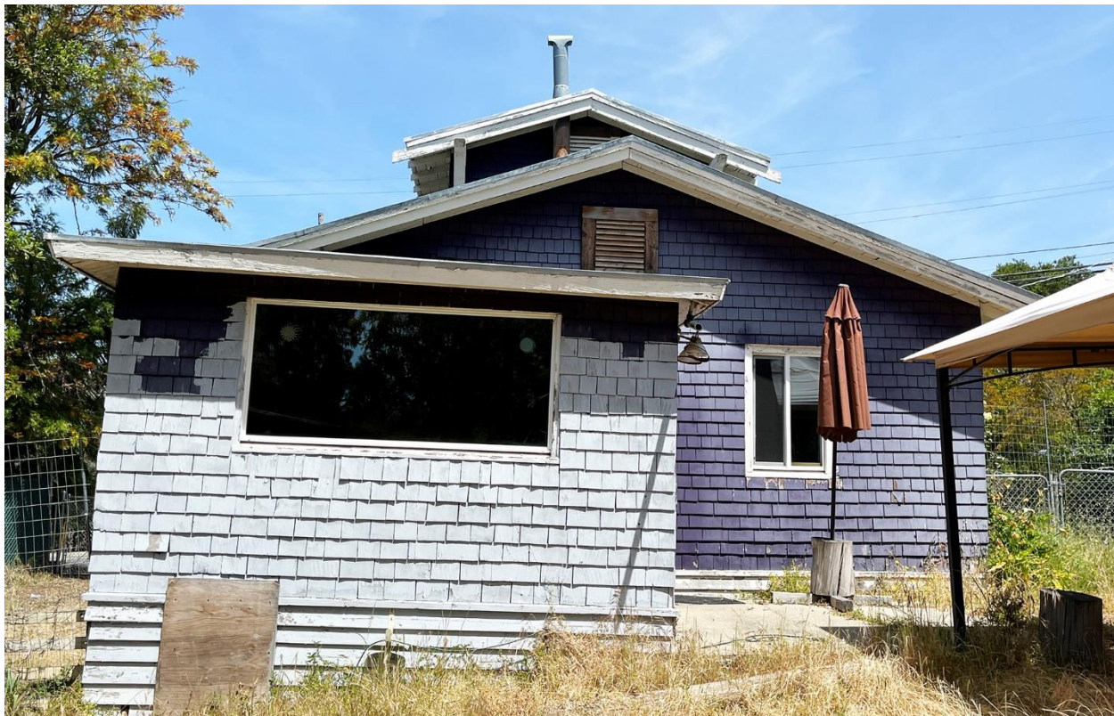
Figure 14. South (rear) façade, looking north.
