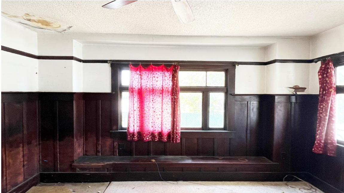
Figure 15. Living room, looking east toward inglenook.
