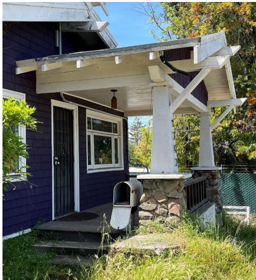
Figure 8. Detail of front porch, looking west.
