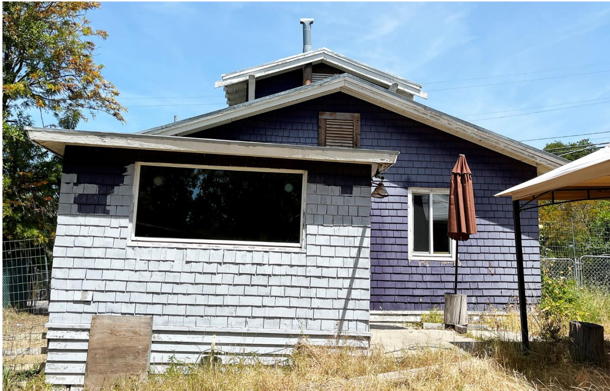
Figure 14. South (rear) façade, looking north.
