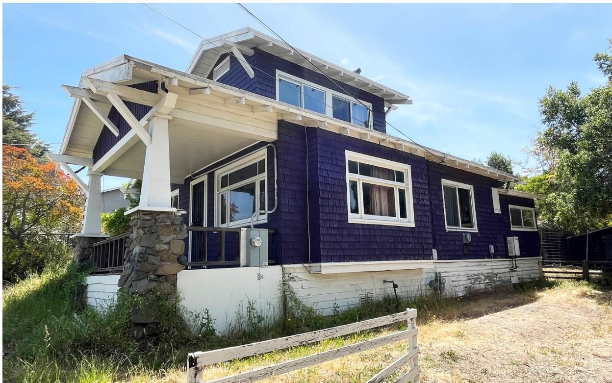
Figure 10. West (secondary) façade, looking southeast.
