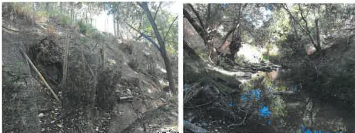
Some steep and unstable banks of San Lorenzo Creek
