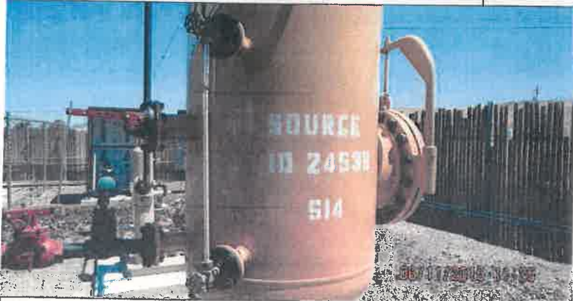
DESCRIPTION: CURRENTLY CLOSED SYSTEM, LEVEL GAUGE IS BROKEN
