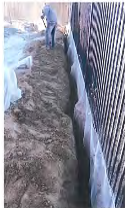
Figure 5.1 Wire mesh barriers to protect from for rodent damage
