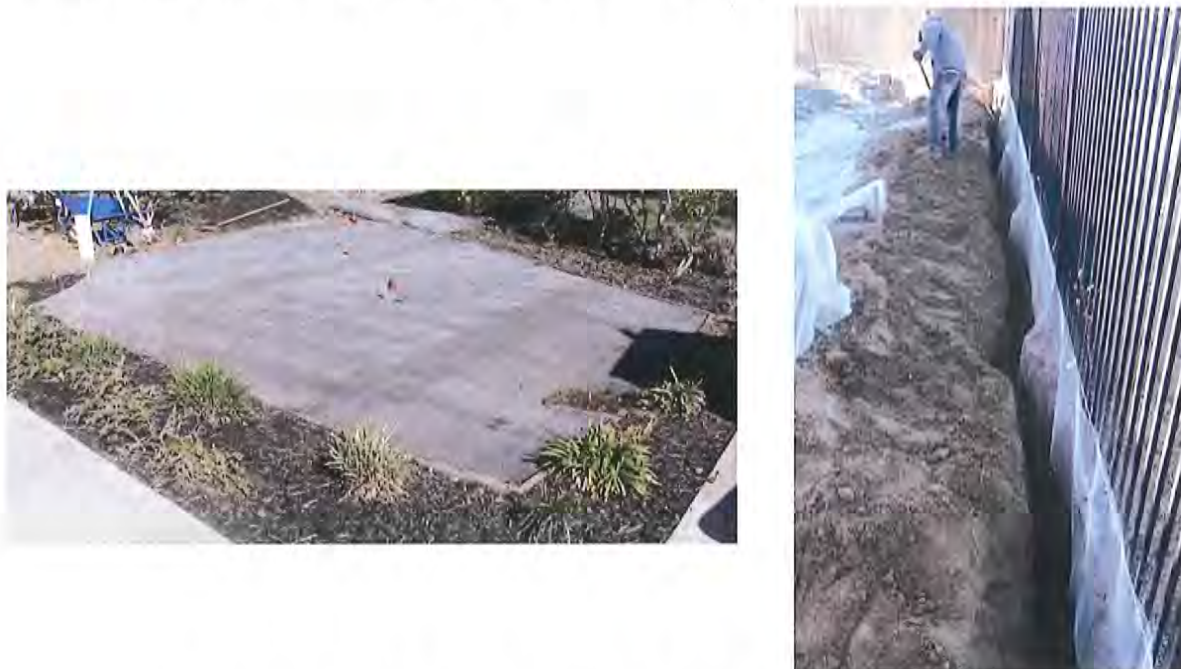
Figure 5.1 Wire mesh barriers to protect from for rodent damage
