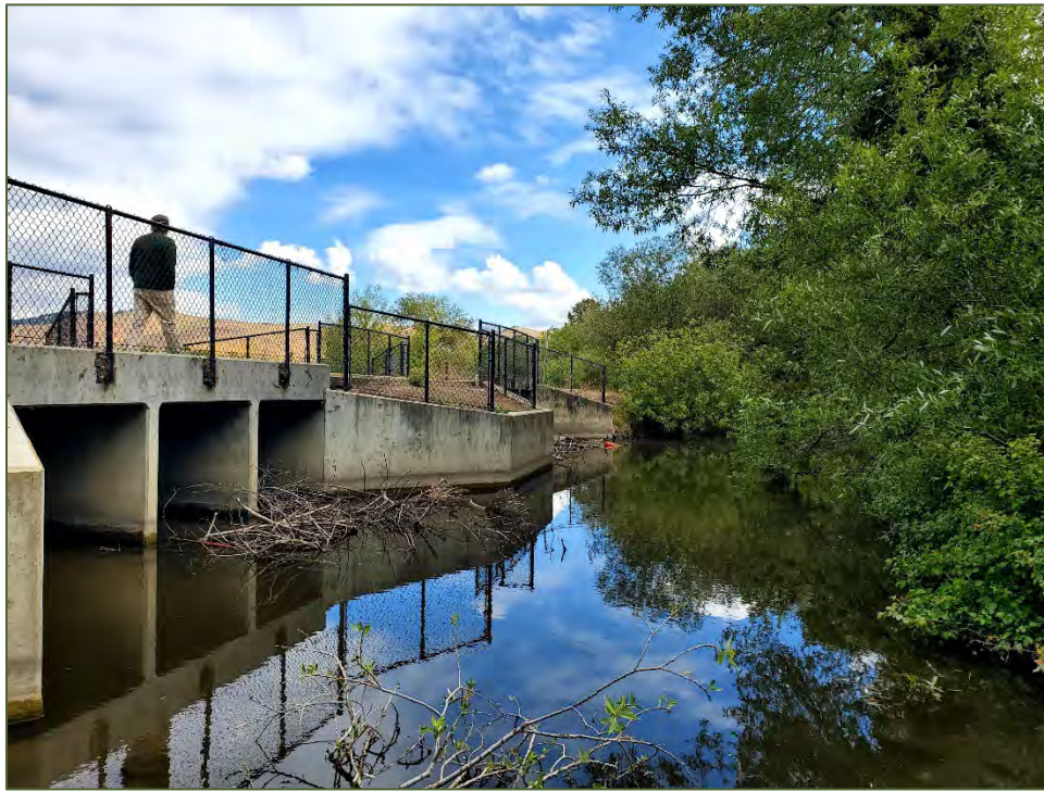
Photo 3. Flapgate and box culvert that connects Lake Elizabeth to Mission Creek with riparian scrub. Facing northeast. April 25, 2022.
