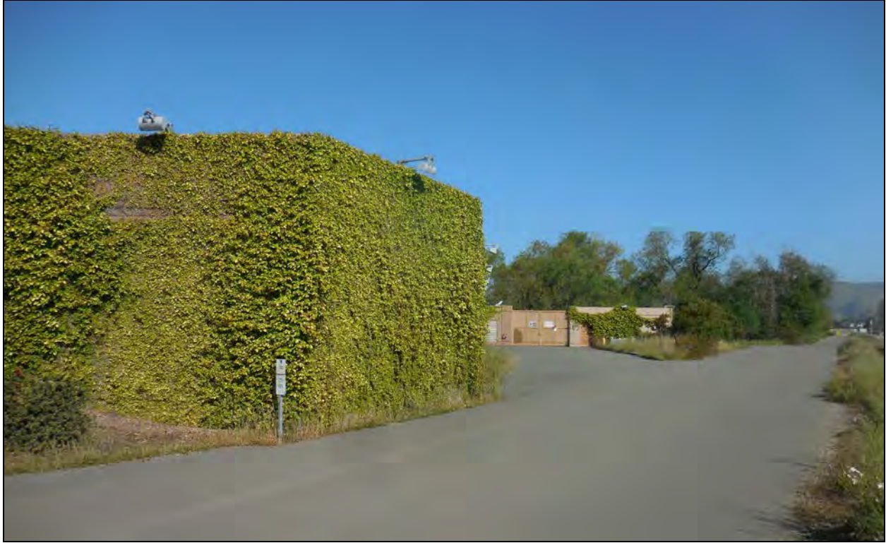
Figure 18: View north towards BART facility (probable ventilation structure – 40690 Paseo Padre Parkway)
