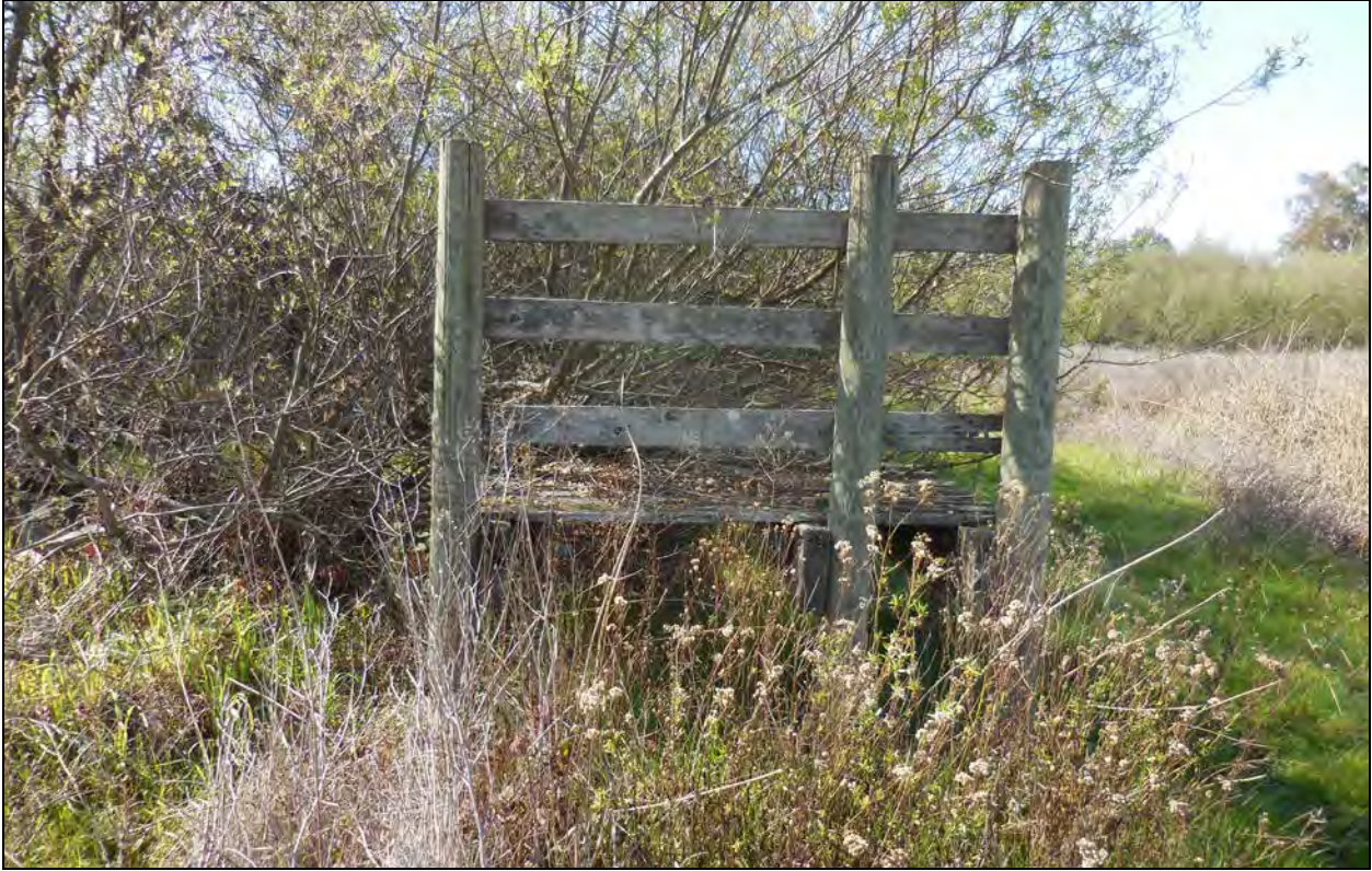
Figure 10: North end of existing catwalk
