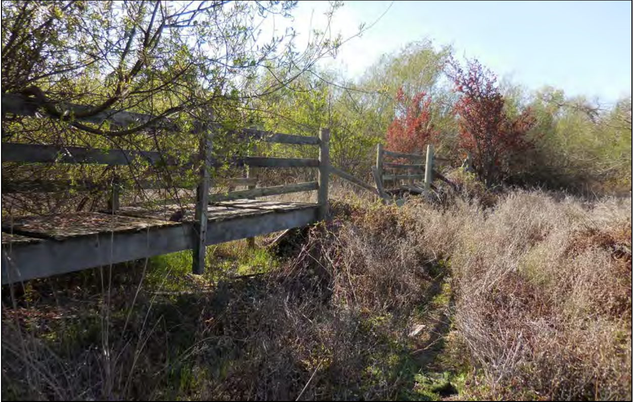
Figure 11: Existing catwalk – view to northwest
