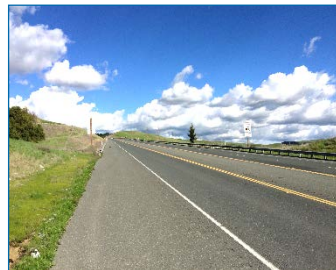
SR-84 looking westbound near Ruby Hill
