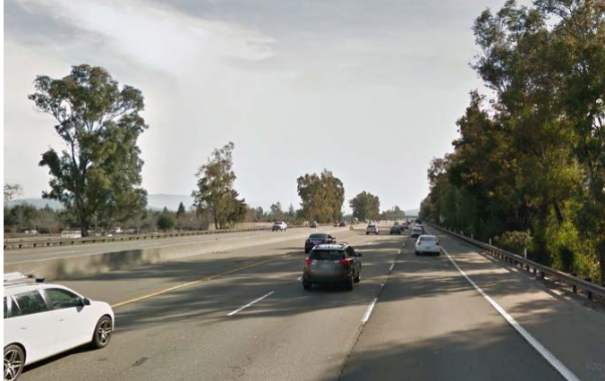
I-680 southbound south of Stoneridge Drive.
