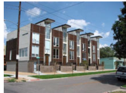
The townhouse units, as well as the project as a whole, do not have an architectural style assigned. It could be contemporary Mission style or a more modern style.
