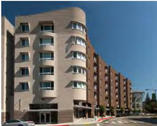
RCD's Oxford Plaza includes 97 units above 8,500 square feet of commercial space, including our office, yoga studio and restaurant. Below grade, the City of Berkeley operates a parking garage including City Car Share Spaces
