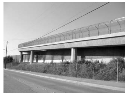
Require noise mitigation measures for projects near I-580.
