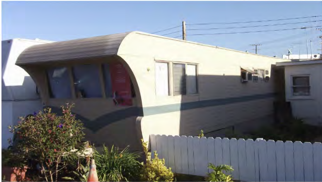
PHOTO 15. 16309 Kent Avenue – Unit 4 Next to Bath Structure at Right
