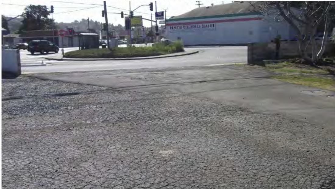
PHOTO 36. 16309 Kent Avenue – Main East Entrance
