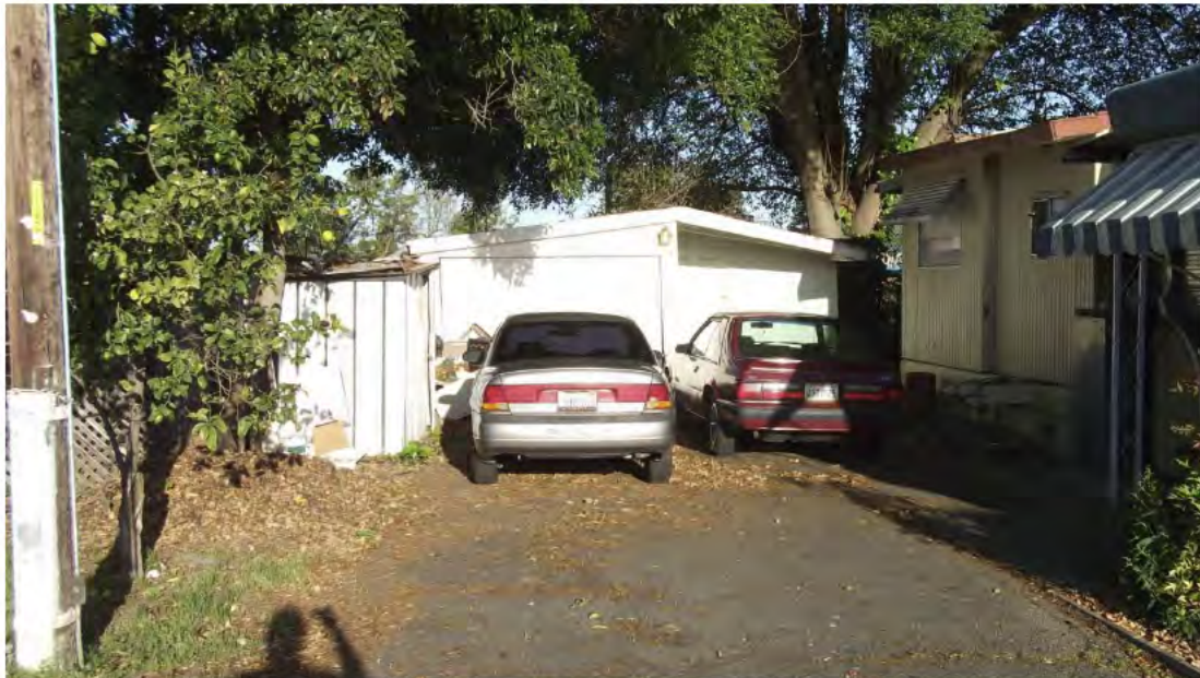
PHOTO 20. 16309 Kent Avenue – Unit 9 Garage Structure with Shed (not accessible)
