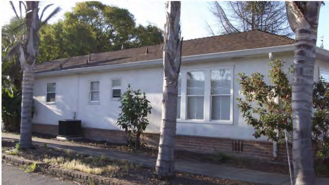
PHOTO 8. 16331 Kent Avenue - Single Family Residence with No Garage
