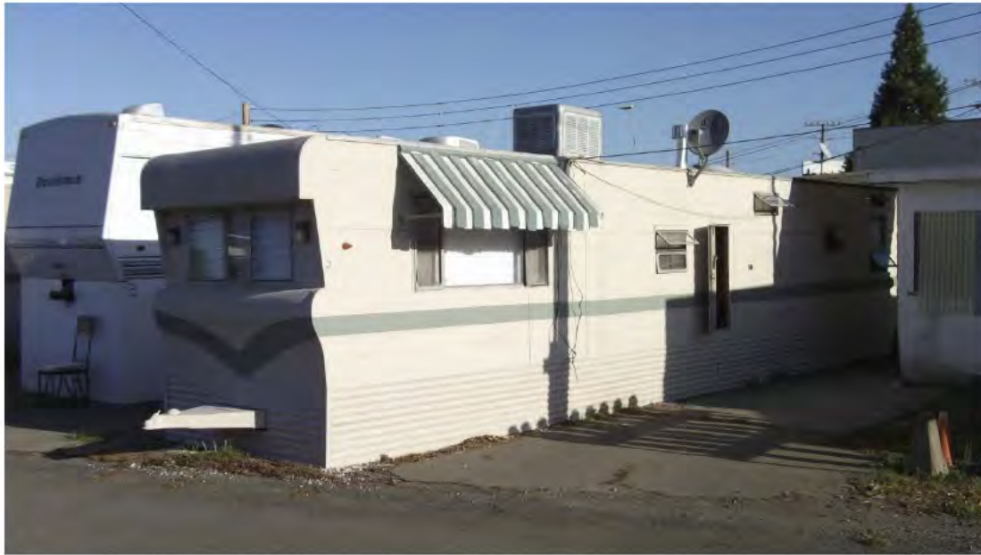
PHOTO 13. 16309 Kent Avenue – Unit 2 Next to Bath Structure at Right
