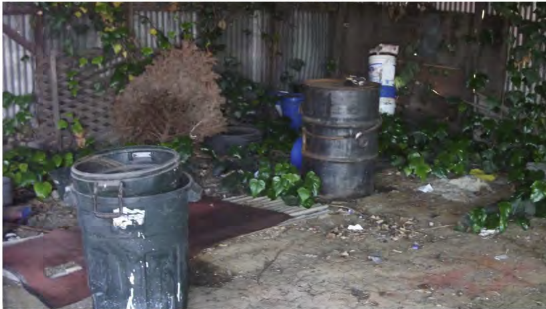
PHOTO 32. 16309 Kent Avenue – 14-car Parking Shed with Discarded Oil Drums
