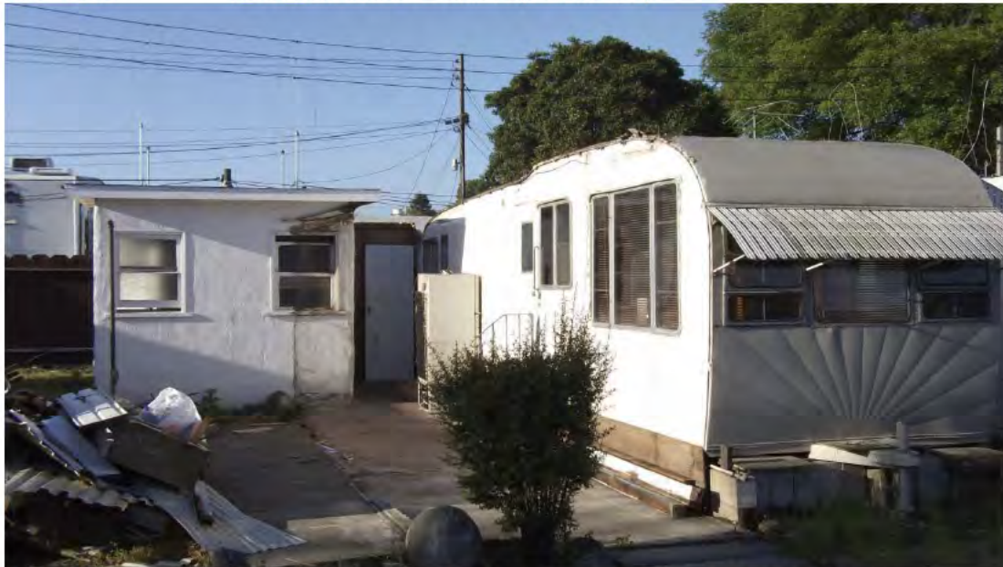
PHOTO 28. 16309 Kent Avenue – Unit 11 (unoccupied) adjacent to Bath Structure
