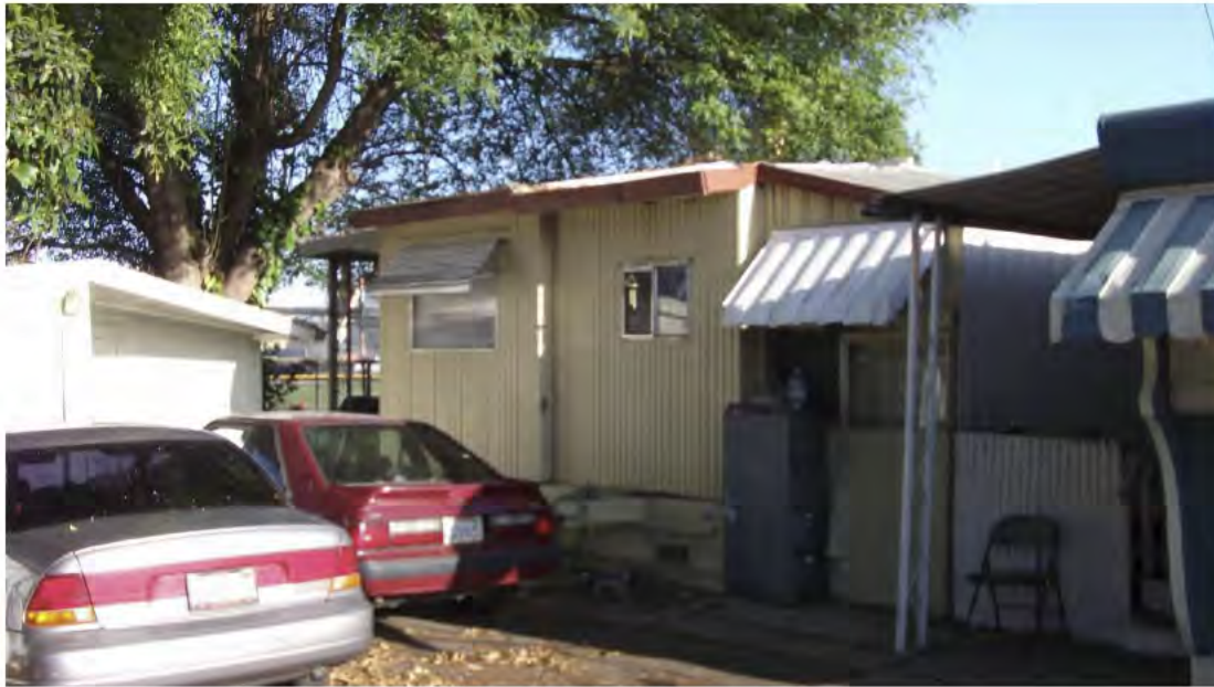
PHOTO 19. 16309 Kent Avenue – Unit 8 Next to Garage Structure (at left)
