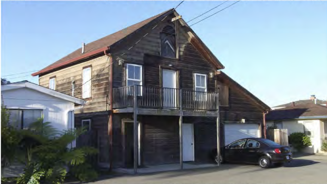
PHOTO 3. Barn - Single Family Residence With One-car Garage Plus Community Laundry
