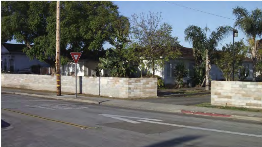
PHOTO 7. 16331 Kent Avenue - Single Family Residence with No Garage
