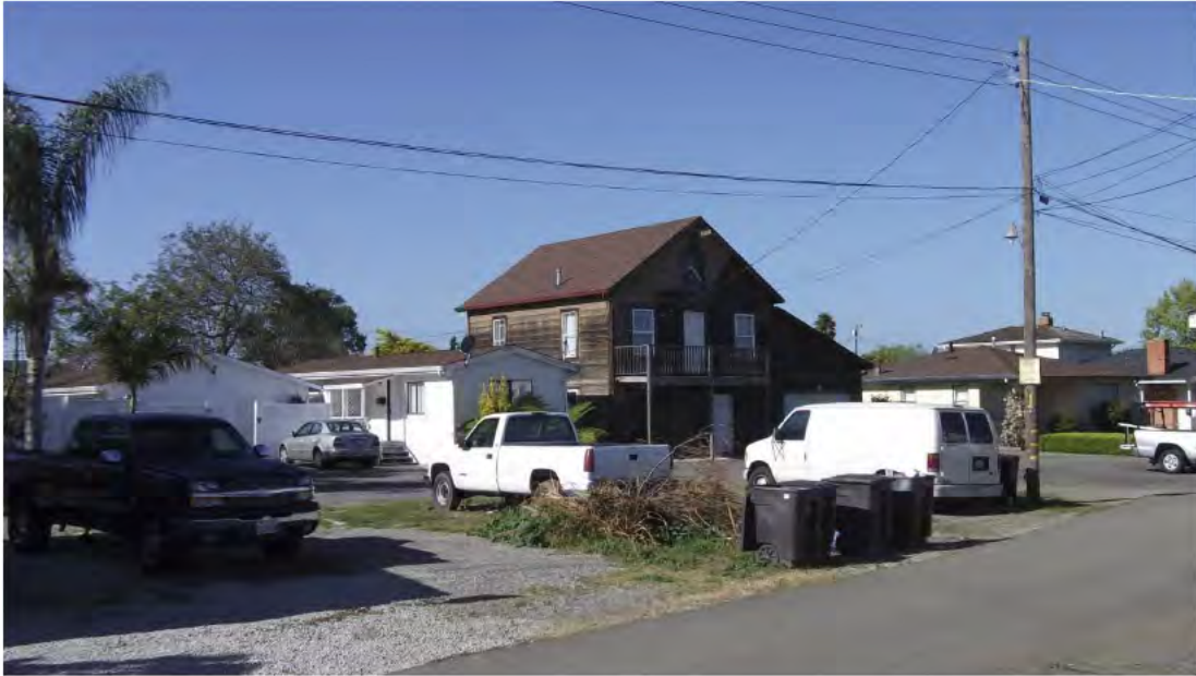
PHOTO 2. Barn - Single Family Residence with One-car Garage plus Community Laundry
