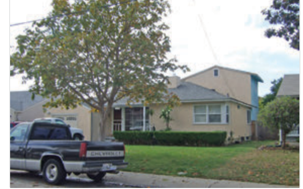
The roof form of the second story addition is not consistent with the existing roof forms and the window is not consistent with the first story windows. (Guideline D-23)
