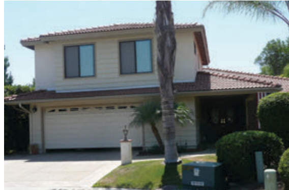
The second story addition has a roof form and roof materials consistent with the first story garage. (Guideline D-23)
