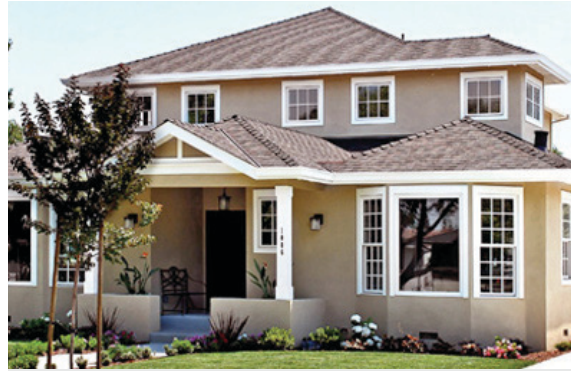
The second story addition is located away from the adjacent property, which minimizes bulk and impacts on adjoining properties. (Guideline D-22)
