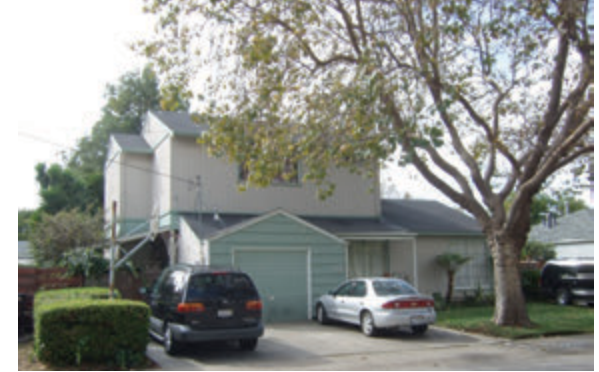
The second story addition does not match the window proportion or siding of the first story. (Guideline D-21)
