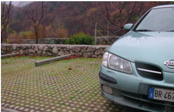
Incorporate innovative stormwater management practices, such as permeable pavers in parking areas. (Guideline J-11)
