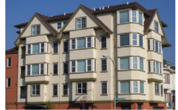
This project uses too many different window designs (different bay window styles, smaller windows are not consistent) which results in an inharmonious facade. (Guideline E-34)
