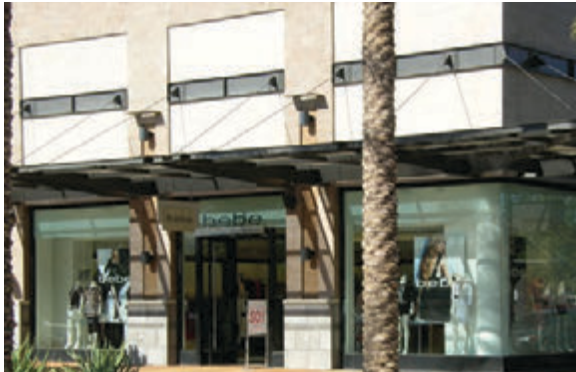
This ground floor storefront consist of clear glass display windows and a glass entry, allowing pedestrians to see inside the space. (Guideline E-4)
