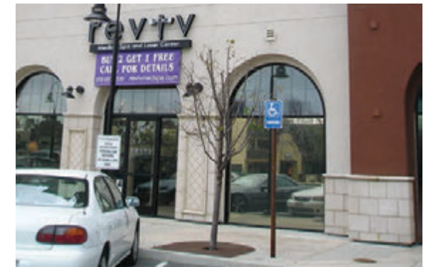
This project uses tile for the first three feet above the sidewalk level, which is highly durable and adds a decorative element to the ground floor design. (Guideline E-7)
