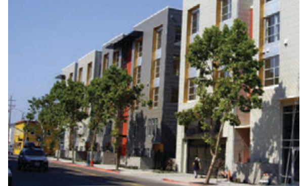
Provide new or repaired improvements in the public right-of-way along the lot frontage, including sidewalks, street trees, curbs, and gutters. (Guideline I-1)
