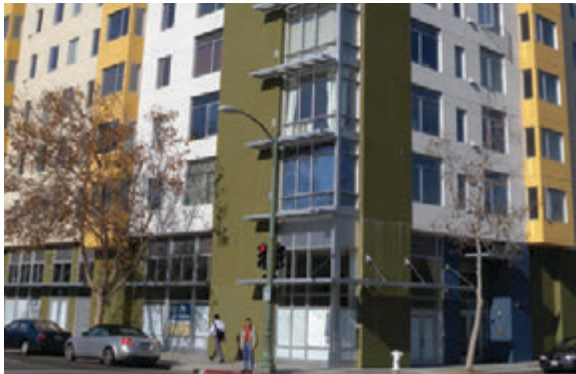
The green and yellow colors on this facade serve as accent colors, rather than being used for the entire facade. (Guideline E-15)
