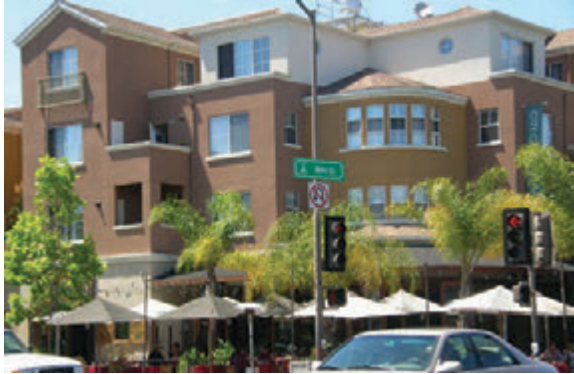
In this project, breaking up the building into smaller discrete masses minimizes the bulk of the building. (Guideline C-5)
