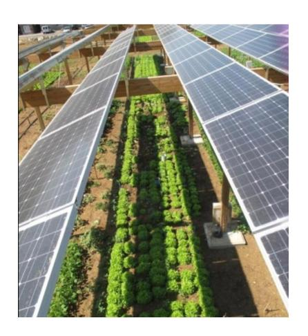
Agrivoltaics (AVs), the co-located production of solar energy and crops, is an emerging technology that can reduce competition for land, and provide climate-smart solutions to improve land use efficiency (combined crop and electricity yield), crop water-use efficiency, profitability and the economic resilience of farmers.
