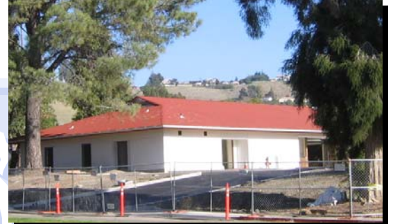
Construction underway on the Safe House sobering center
