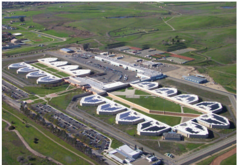
Solar Installation at the Santa Rita Jail consists of nearly 3 acres of Power-Light's roof top PV tiles.
