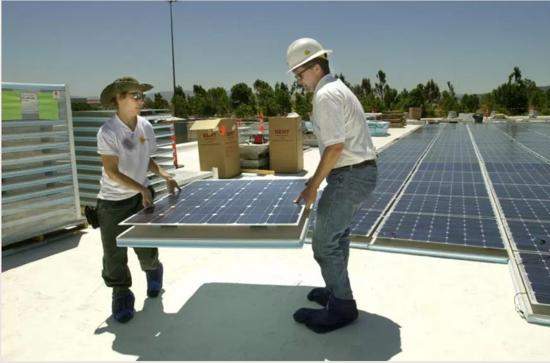
Workers install photovoltaic panels on the roof of the county's Santa Rita Jail in 2001. (Dan Honda/Bay Area News Group)
