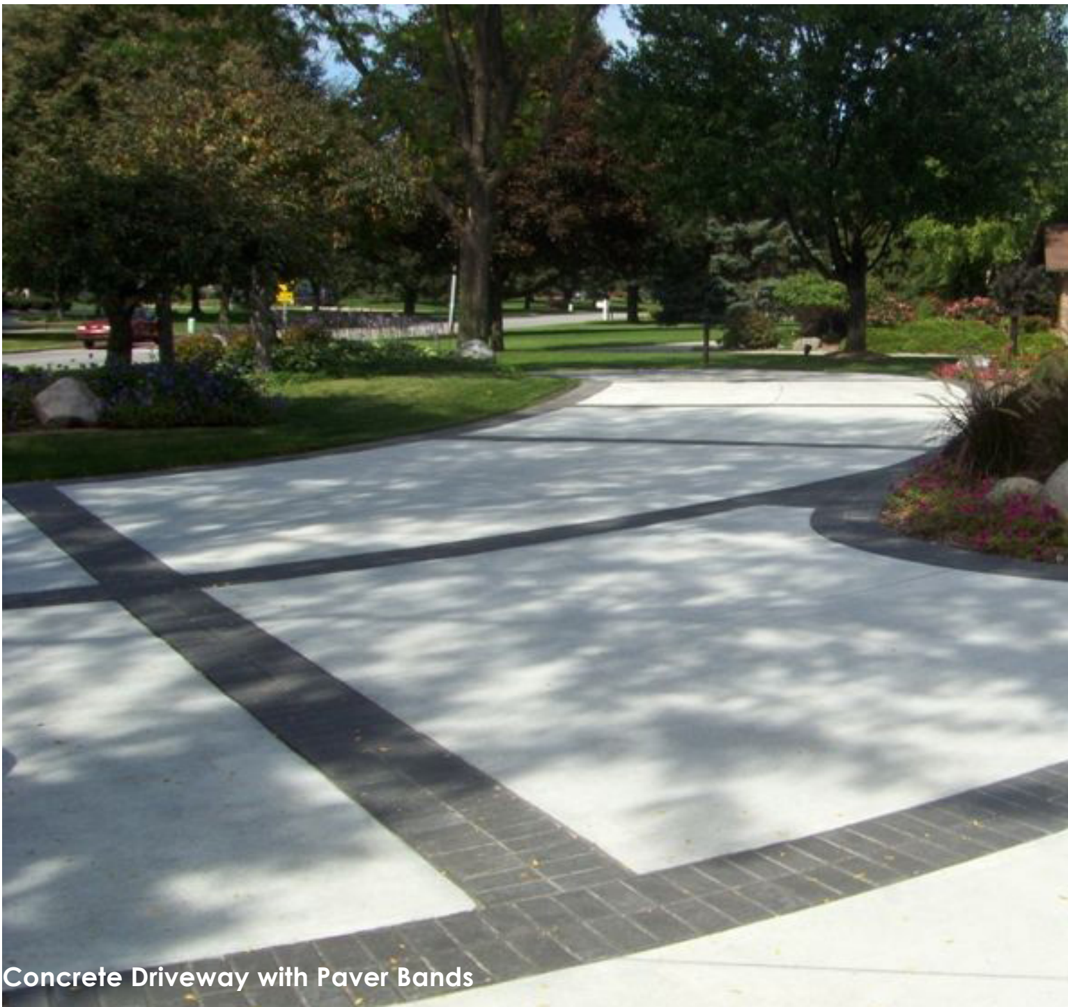
Concrete Driveway with Paver Bands
