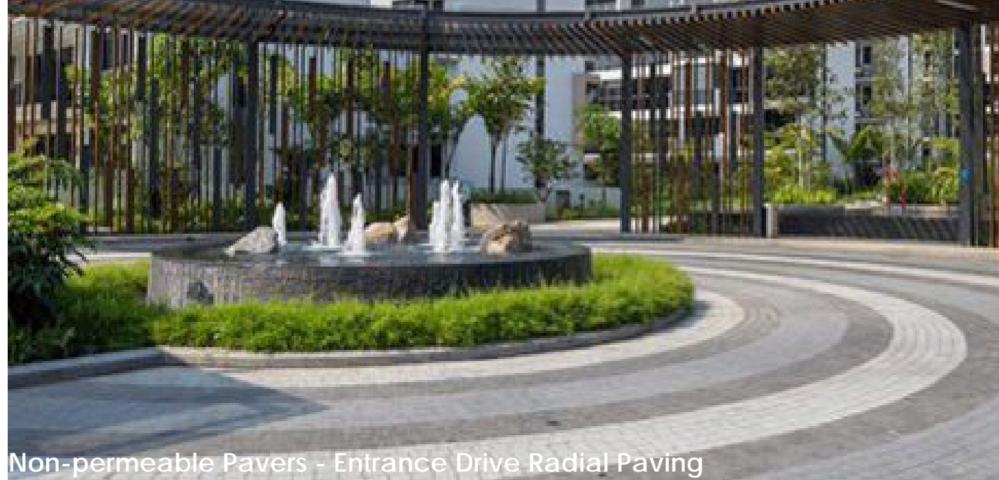
Non-permeable Pavers - Entrance Drive Radial Paving
