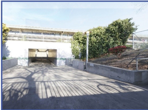
Bay Fair BART Station Tunnel Existing Condition - County Side
