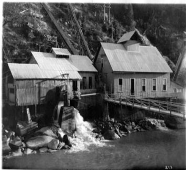
Rome/Rome Power House on South Yuba River
