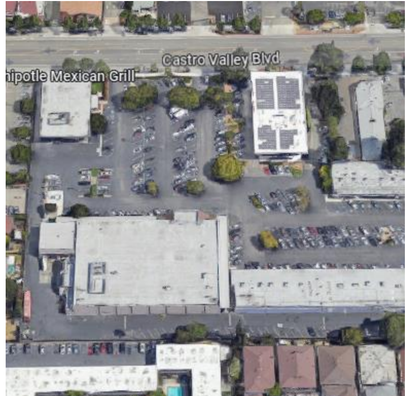
Figure B-5. Lucky's Parking Lot
