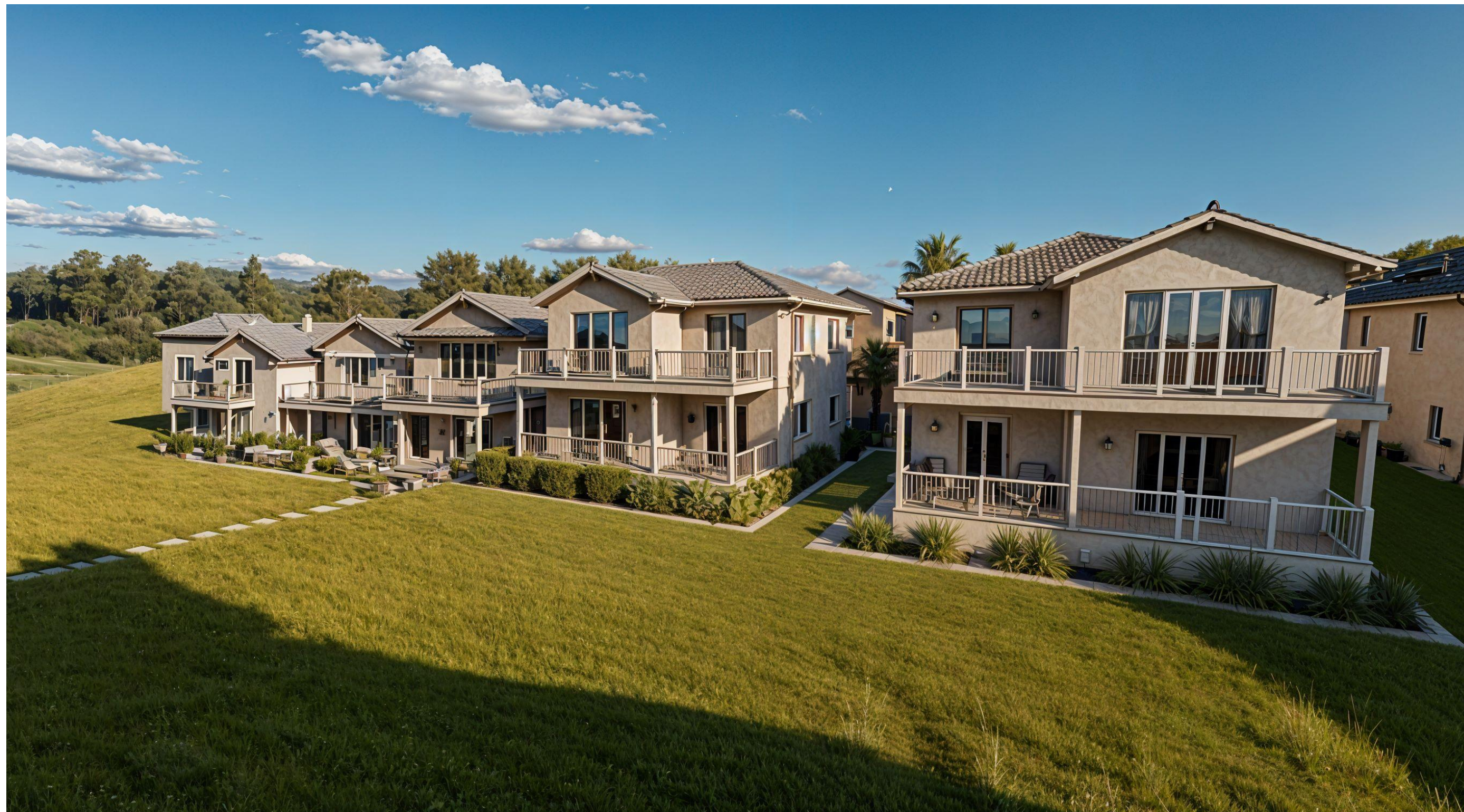
DOWNSLOPE REAR OF HOMES.
