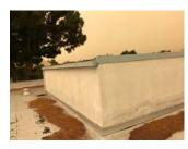
19. Replace stucco where Building C and B meet to make joint watertight.
