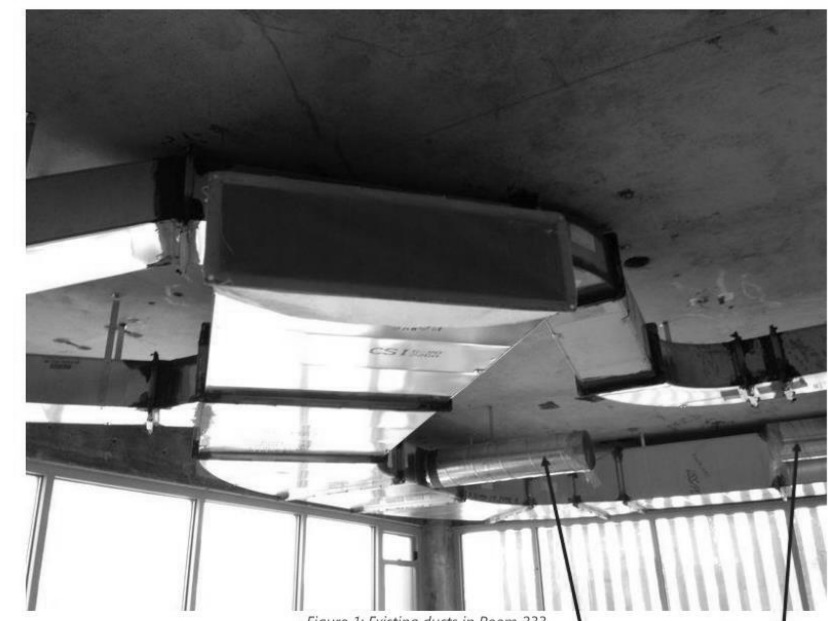
Figure 1: Existing ducts in Room 233
