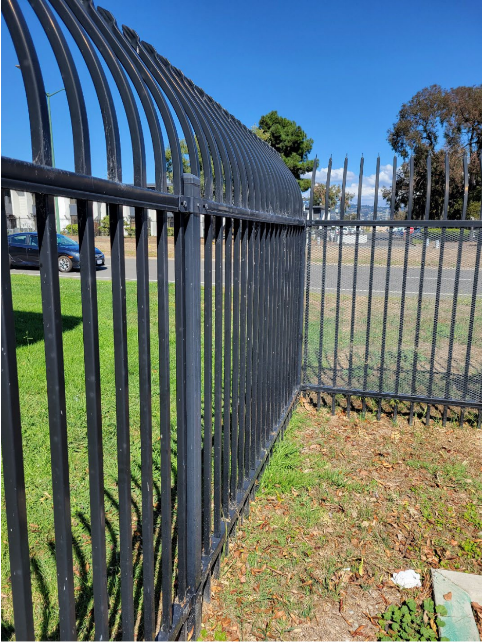
Typical fence panel. Shown for design purposes, construction to be per specifications.
