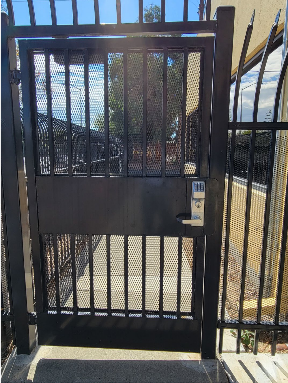
Typical exterior view with trilogy lock. Incorrect lock shown. Specified lock is trilogy 2700WP.
