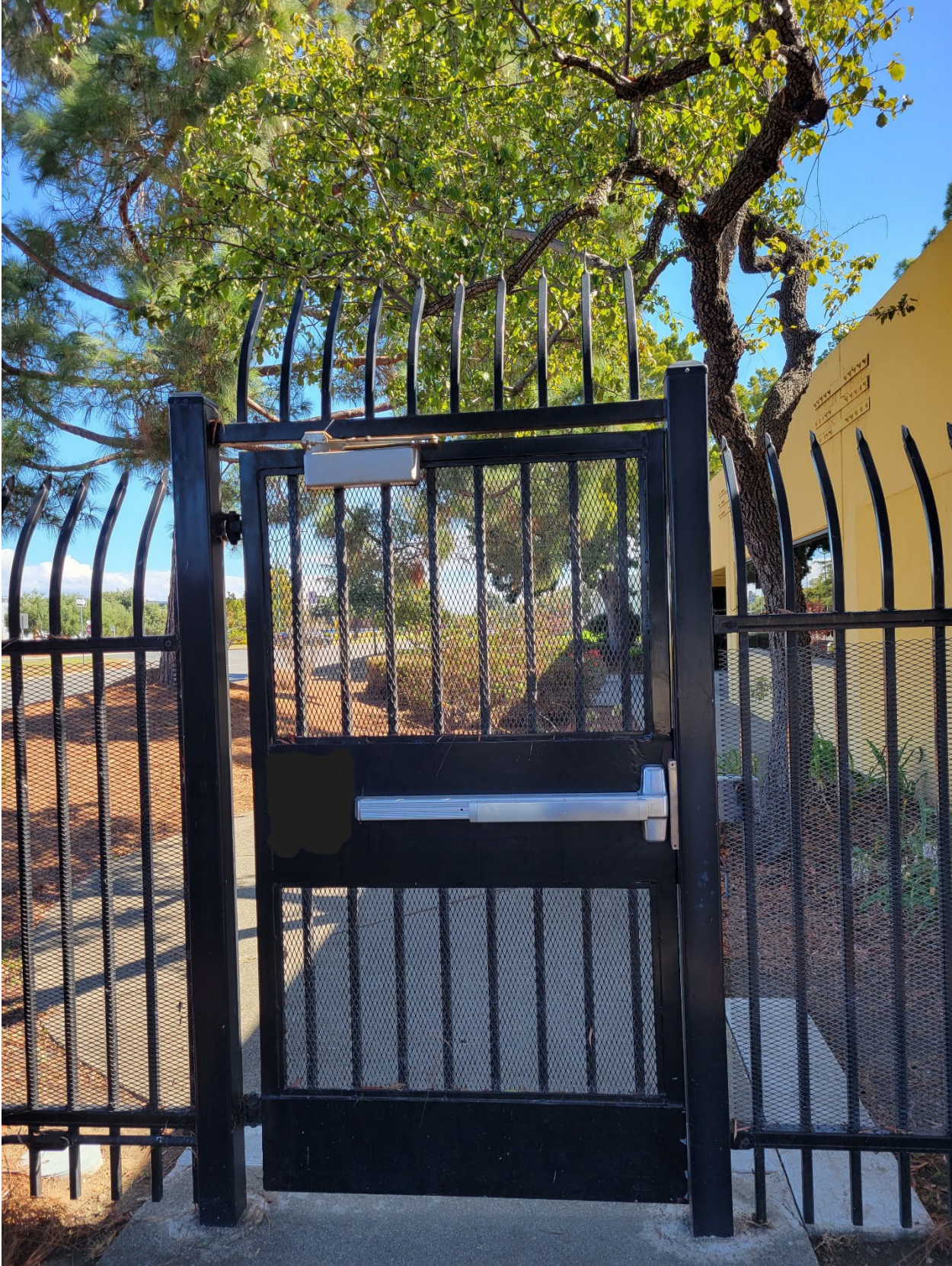
Typical gate, interior. Note mesh.
