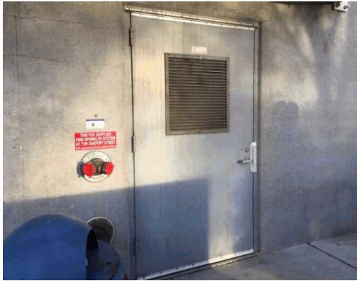
Item #: 489170 Uniformat Number: B2050 Item Title: Exterior Doors And Grilles Caption: Exterior Door 1 Priority: 3 - Necessary - Not Yet Critical
