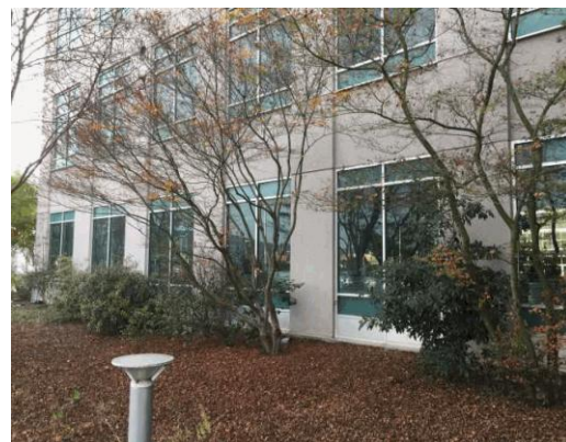
Item #: 490022 Uniformat Number: B2020 Item Title: Exterior Windows Caption: Exterior windows on facade 2 Priority: 2 - Potentially Critical
