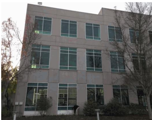
Item #: 490022 Uniformat Number: B2020 Item Title: Exterior Windows Caption: Exterior windows on facade Priority: 2 - Potentially Critical
