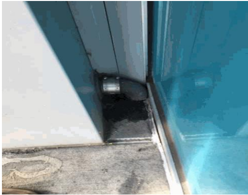
Item #: 491219 Uniformat Number: B3020 Item Title: Downspouts Caption: Downspout at exterior Priority: 2 - Potentially Critical
