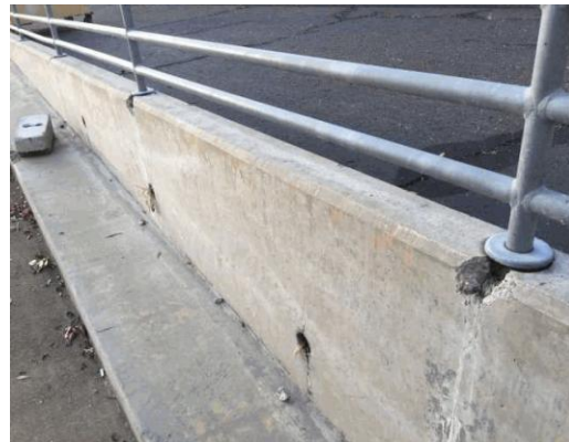
Item #: 489215 Uniformat Number: G2030 Item Title: Exterior Concrete Ramps Caption: Concrete wall at loading dock ramp 2 Priority: 2 - Potentially Critical
