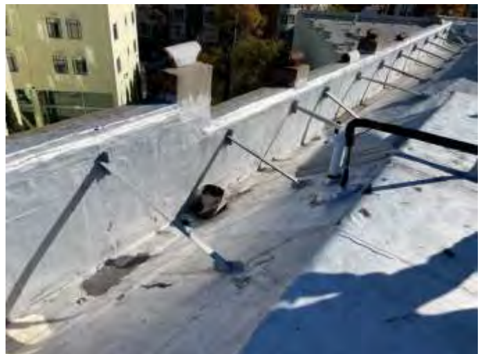
18. Parapet wall bracing
