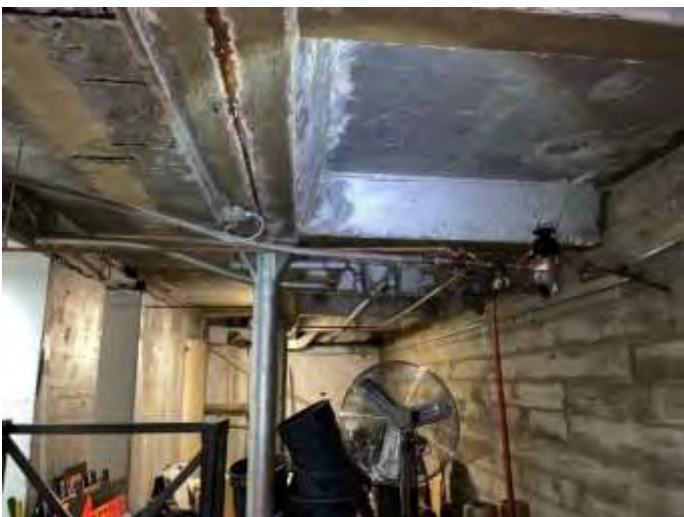
9. Concrete at perimeter of basement
