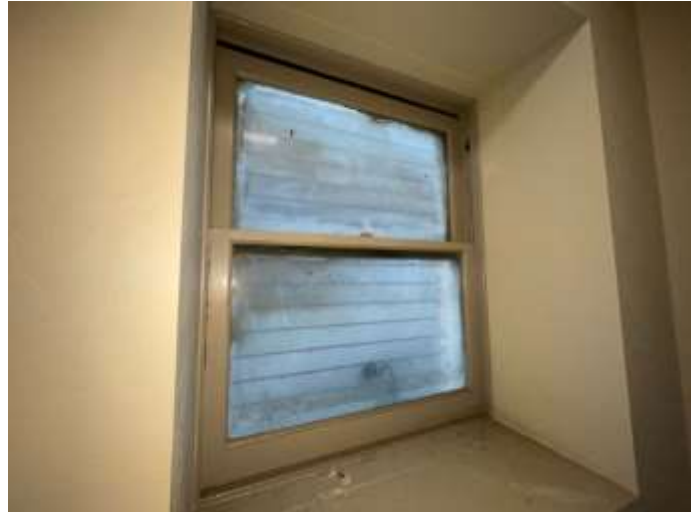
14. Typical wood framed exterior window
