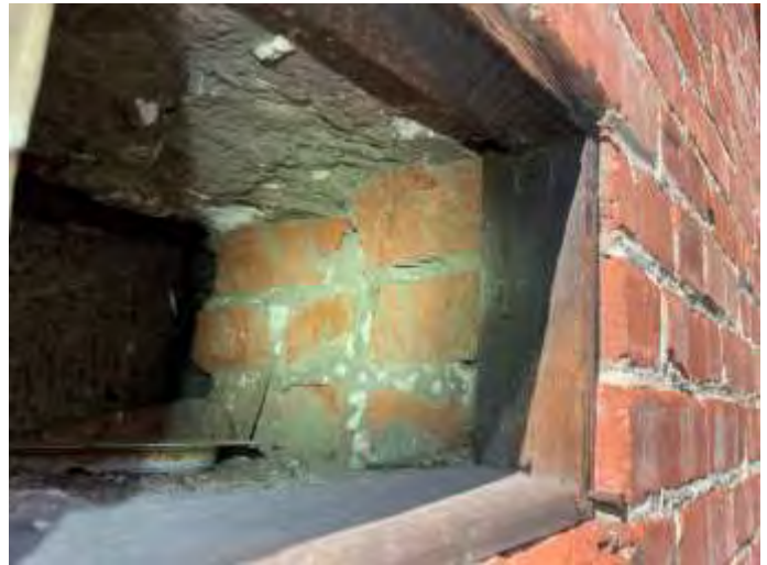
8. Four wythe wide brick at ground level
