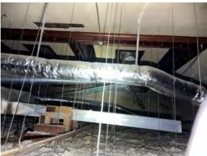
11. Two ceiling systems above the auditorium
