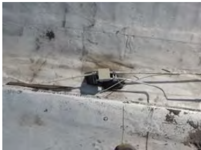
94. Junction box positioned within stormwater discharge path
