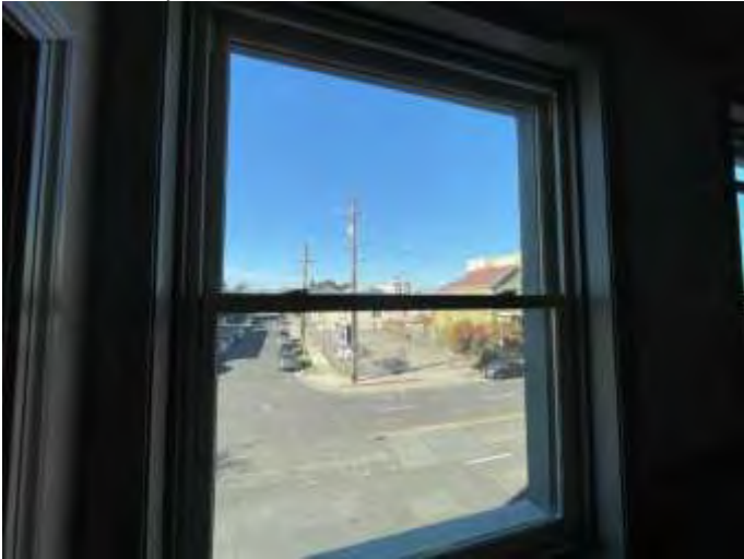
13. Typical aluminum framed exterior window
