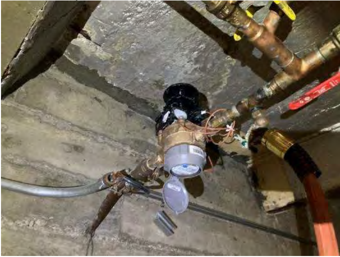
25. Water service entrance in the basement
