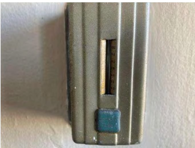
47. Decommissioned mercury thermostat
