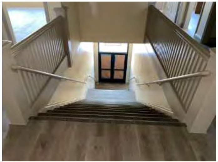
22. Main interior wood stairway to upper floors
