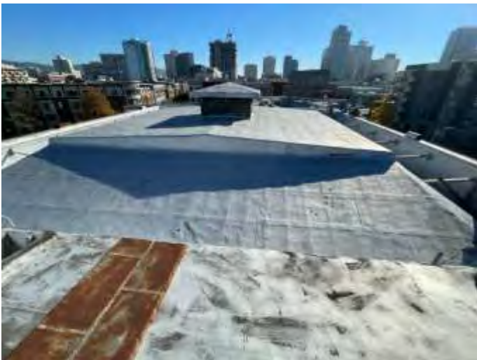
15. BUR with aluminized emulsion coating
