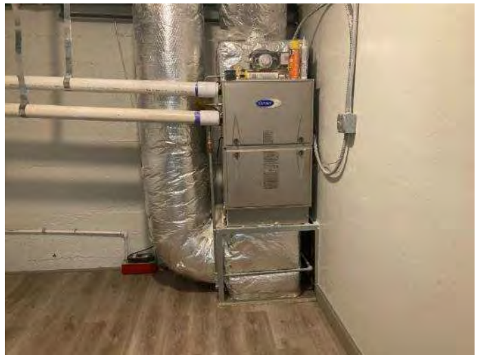
40. Typical condensing gas furnace unit
