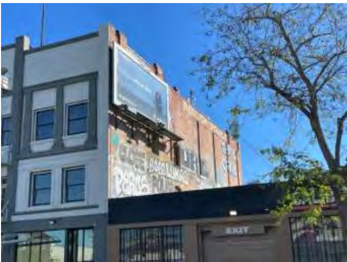
3. South elevation of subject property
