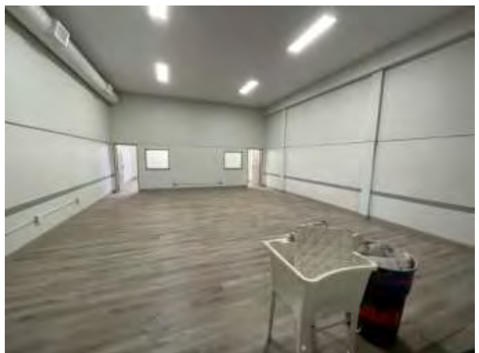
72. Back room on ground floor with 1x1 acoustic tile walls
