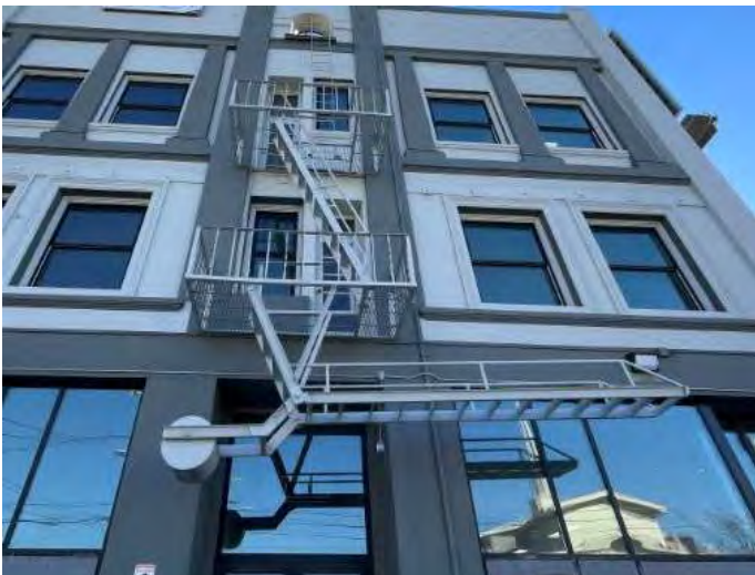
21. Steel fire escape on front elevation with water tank counterbalance ladder/stairs
