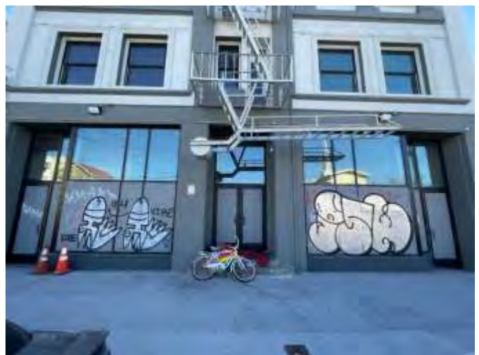
12. Three entrances at front elevation
