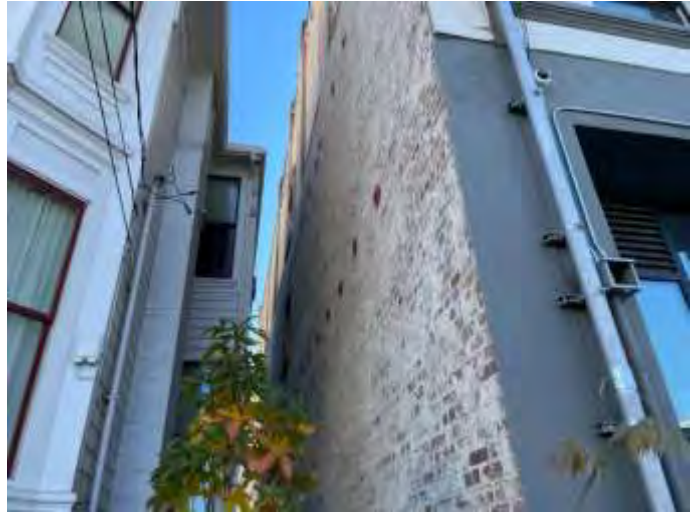
2. North elevation of subject property
