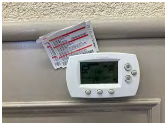
46. Programmable thermostat
