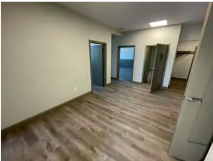
69. Typical hallway finishes
