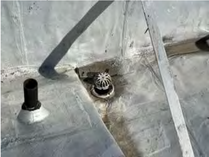
19. Internal drain
