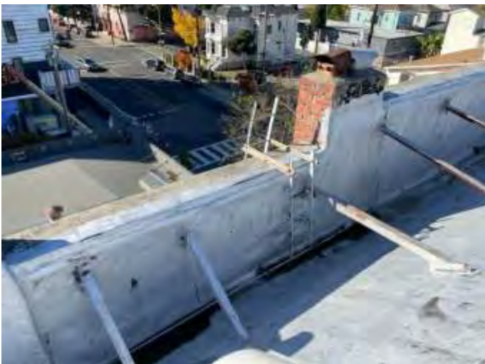
17. Two wythe wide parapet walls
