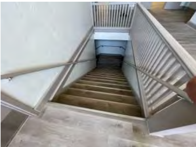
23. Wood stairway to basement
