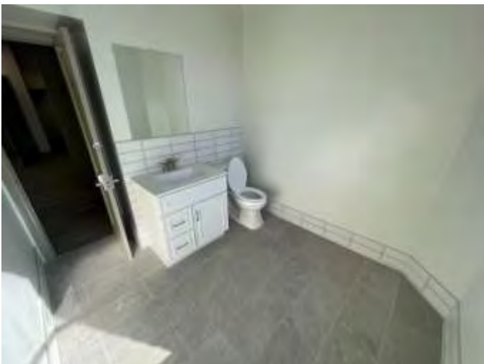
77. Typical upper-level restroom finishes
