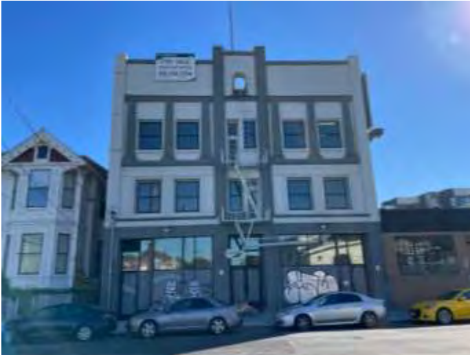
1. Front elevation of subject property
