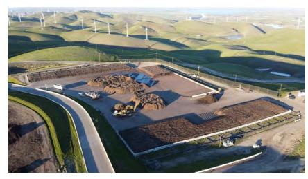
The Altamont Landfill operates a composting facility in Alameda County that converts up to 500 tons of organic waste per day into usable compost to support healthy soil.
