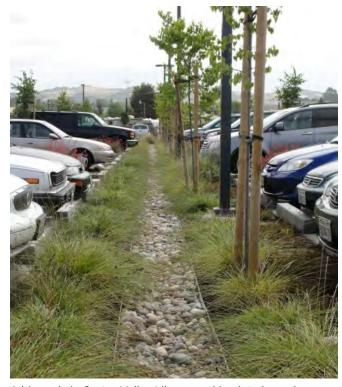
A bioswale in Castro Valley Library parking lot channels stormwater to remove pollution, reduce runoff, and allow water to absorb into the ground.
